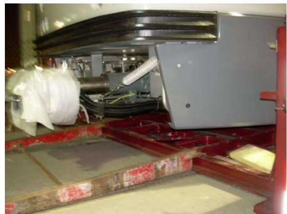
Brake system is released; rear cable wench slowly rolls off P2550 / 705 onto the track.
